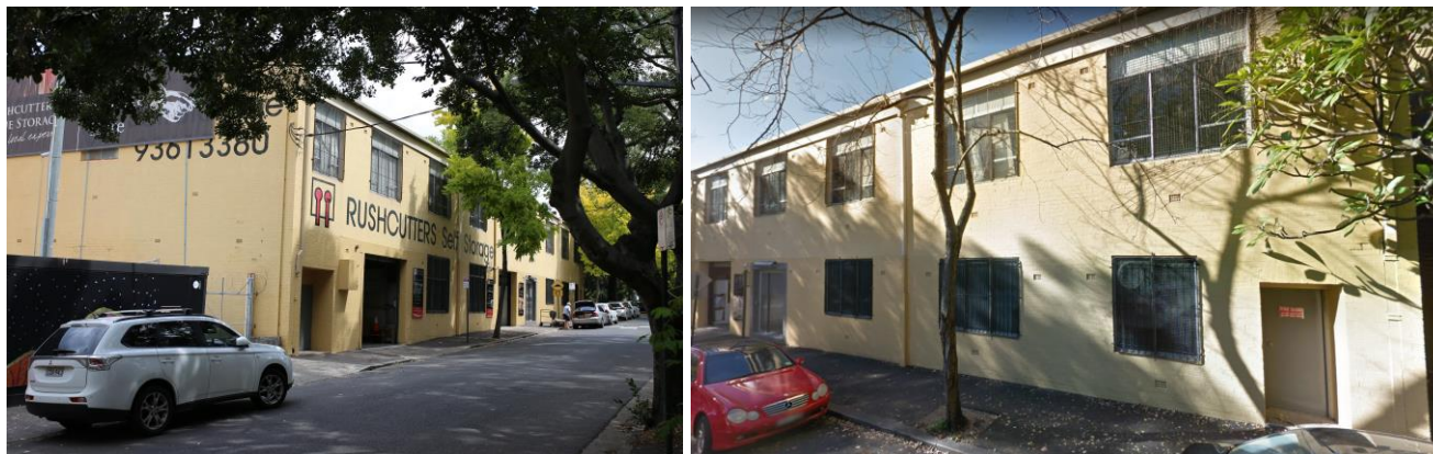
30-62 Barcom Avenue, looking south
