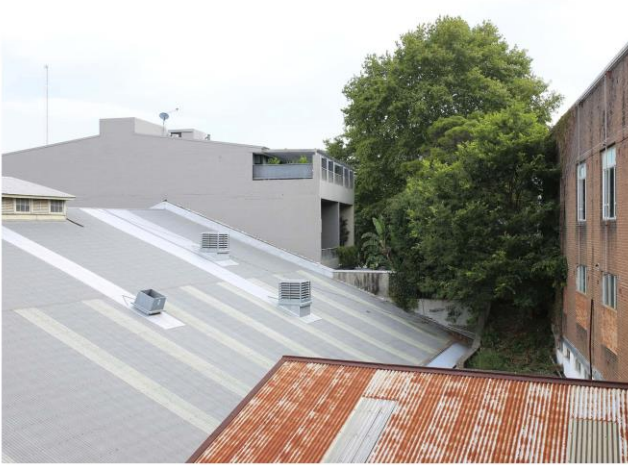
View from 3-062 Barcom Avenue, looking south to residential interface
