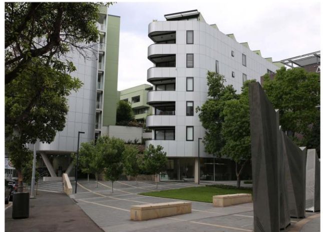
View of mixed use development, plaza and commercial showroom at McLachlan Avenue, looking east
